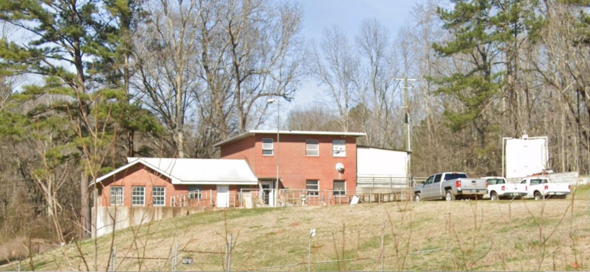
USGS Gage Location 200 Feet upstream of intake
