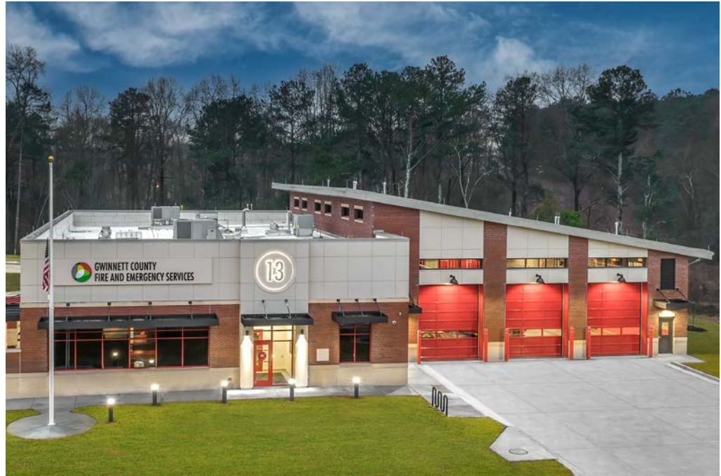
GWINNETT COUNTY FIRE STATION 13 - SUWANEE, GA
