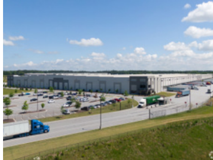
Smuckers Distribution Center
